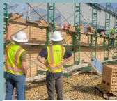
Phase 5: Fulton Middle School Conference and Classroom Additions
